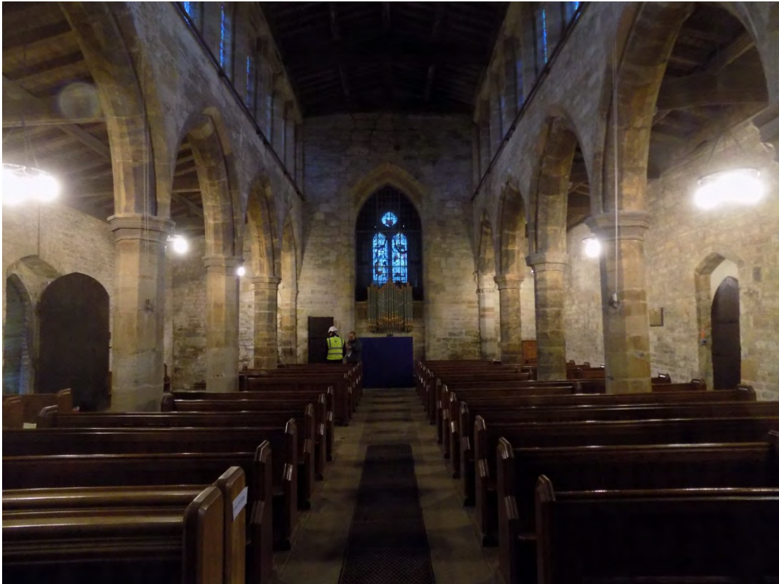
Church nave and aisles (pre-alterations), facing west Fig 5
