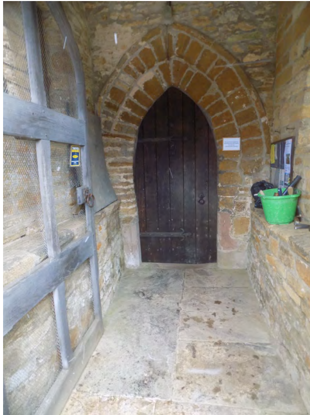
South porch entrance (pre-excavation), facing north
