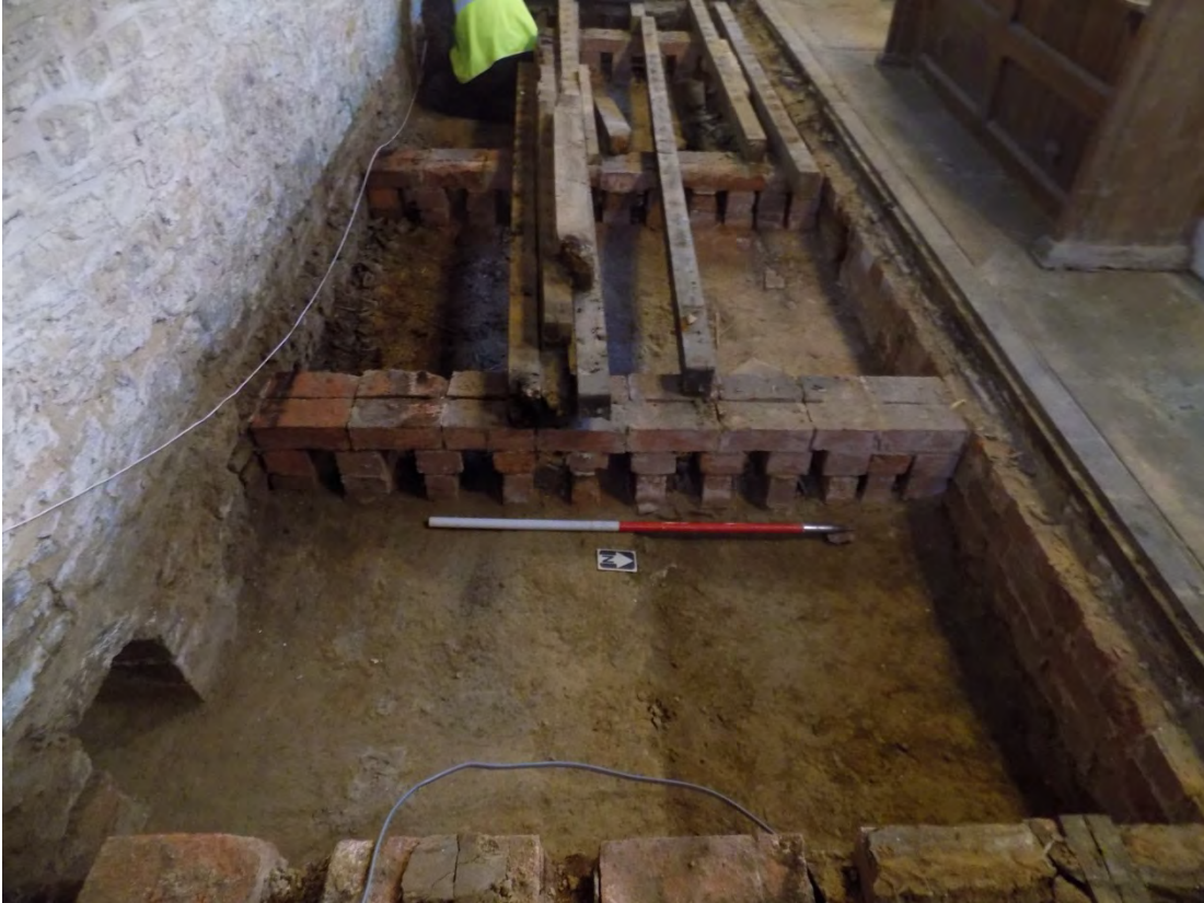
Bay 5, south aisle and brick bay wall (right), floor joist slots visible in brickwork (foreground), nave wall with vent cut (left), dividing brick piers (mid-ground to background) Trench 2 (right, foreground), looking west Fig 22
